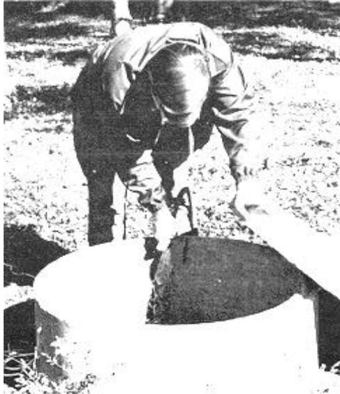
Fig. 3. Strong chlorine solution is recirculated back to the well.
